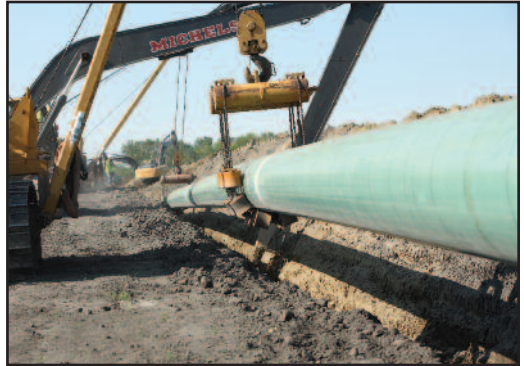
Michels performs work during construction of TransCanada's Keystone Pipeline.
