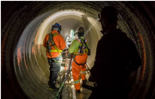
16th Avenue Sanitary Sewer Pilot Study Location: Markham, ON (Canada) Year: 2017
