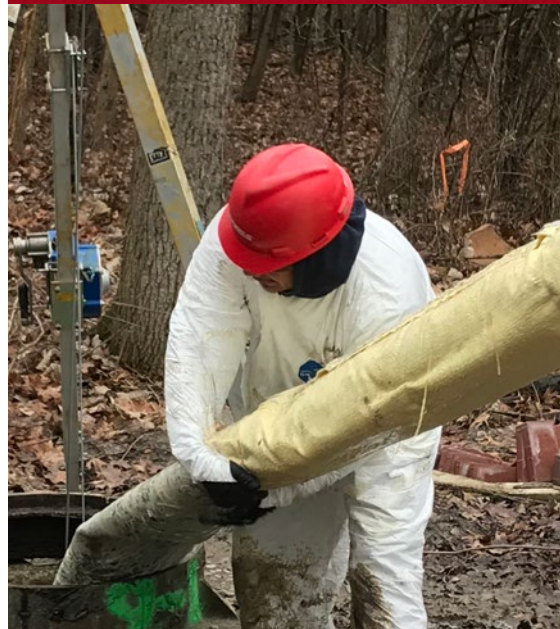
Figure 1: Ambient cured sectional repairs are installed using trenchless technologies, eliminating the need to dig and replace pipe.
