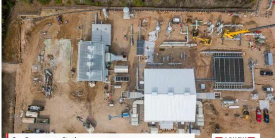
**Gas Compressor Station** Brownfield Suring, WI Complex brownfield compressor station construction on 1 1/2-acre site with groundwater level 2 feet below the surface
